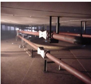
Roof Drain, Pivoted Joint
