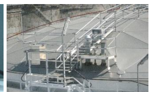
Dome Roof Walkway and Stairs
