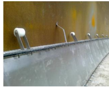
Secondary Roller Wiper Seal
