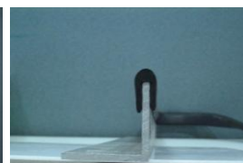
Lip Seal for Manholes Roof Compartments
