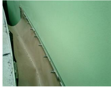
Primary "Y" Scissors Mechanical Shoe Seal
