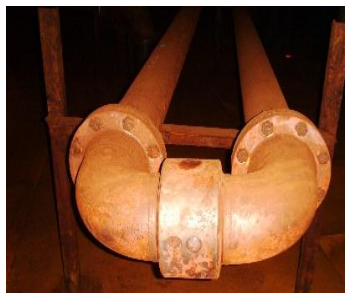
Roof Drain, Swivel Joint
