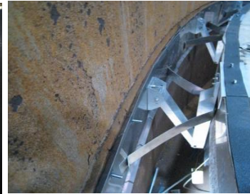
Light Weight Mechanical Shoe Seal
