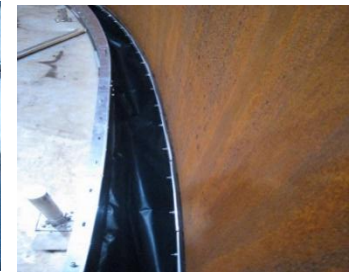
Light Weight Mechanical Shoe Seal
