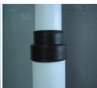
Leg Cup Seal for Roof Legs
