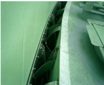
Primary "Y" Scissors Mechanical Shoe Seal
